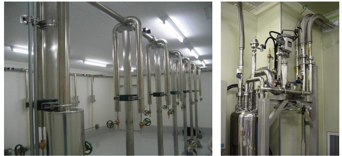
Vacuum Jacketed Piping (Liquid/Gas Separator)
